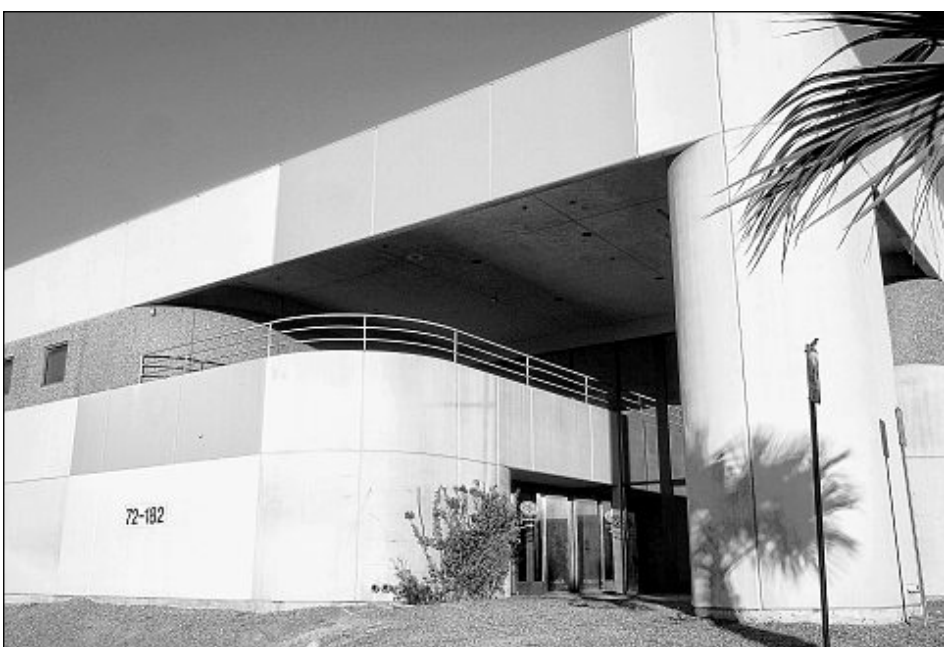
This structure at 72-182 Corporate Way in Thousand Palms, inside the Coachella Valley Enterprise Zone, is the new home of the Tala Enterprise warehouse, with a workforce of 31. RICHARD LUI/THE DESERT SUN
