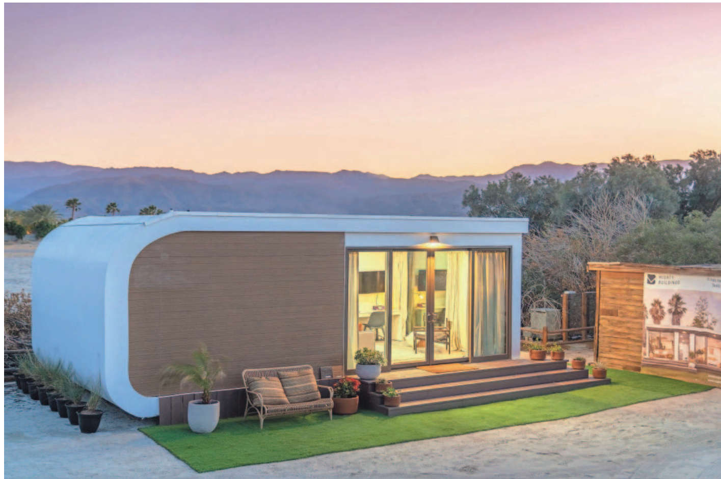
A 3D printed display unit was set up by Palari and Mighty Buildings at the site of the planned 3D printed housing community in Rancho Mirage. The unit has since “closed,” according to Palari CEO Basil Starr.
