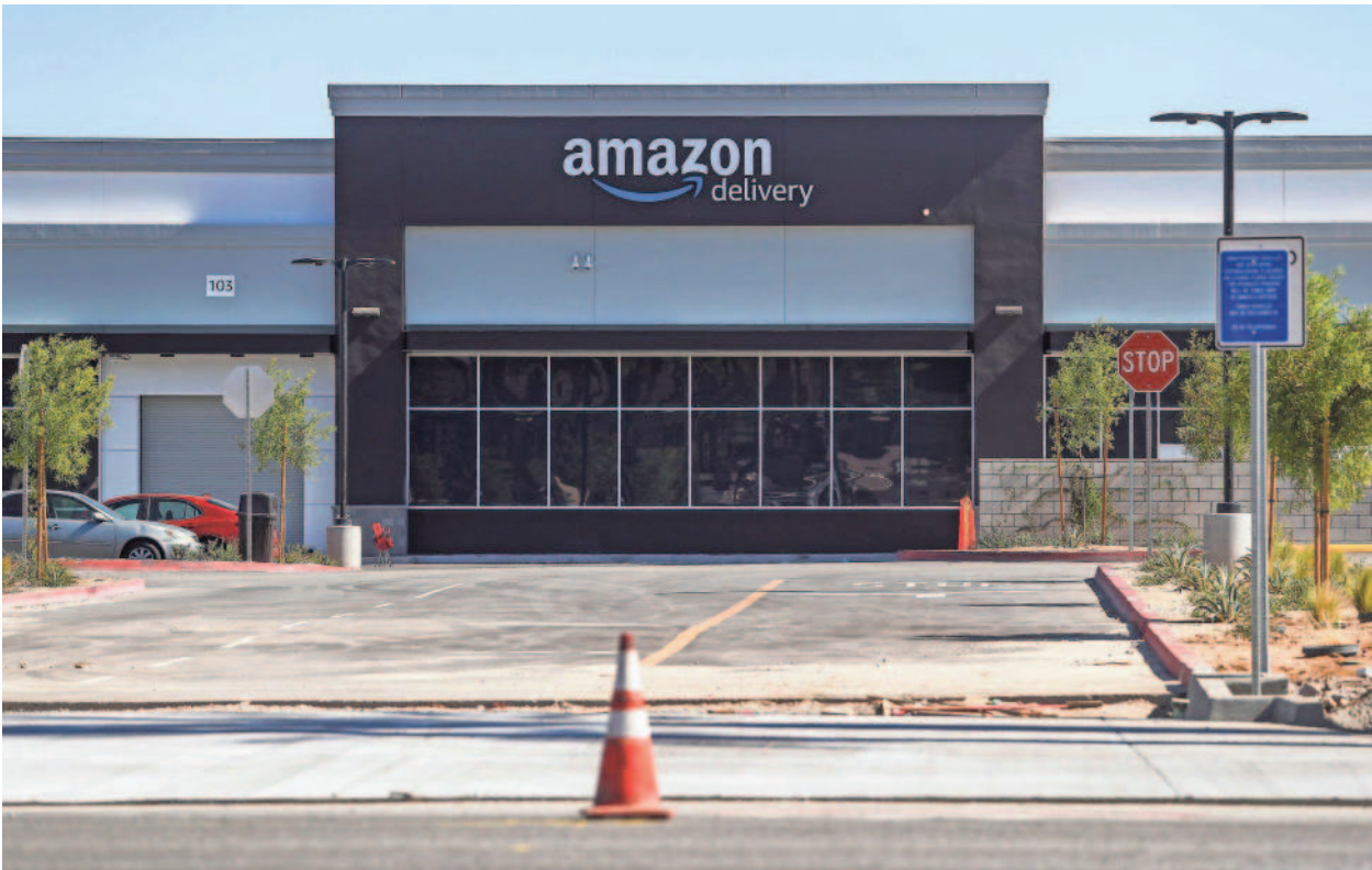
An Amazon fulfillment center is seen under construction at 35800 Date Palm Drive on Tuesday in Cathedral City. The $40 million project occupies a former Sam's Club building that has been vacant for 16 years.
