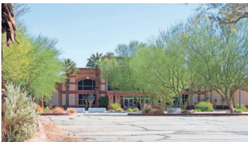
This is the former Burlington Coat Factory building on Date Palm Drive and Gerald Ford Drive on Wednesday. The site has sat empty for nearly four years after the big-box retailer left in early 2018.
