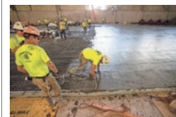
LaRusso Concrete employees pour and smooth concrete for the new iceplex at Acrisure Arena in Thousand Palms on Thursday. The arena may have its first events in December. TAYIA GRAY/THE DESERT SUN
