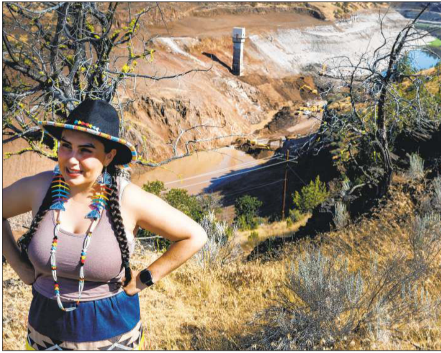
BROOK THOMPSON of the Yurok Tribe stands above the Iron Gate Dam removal site. “It’s like a magic trick, like it was there and now it’s not.”
